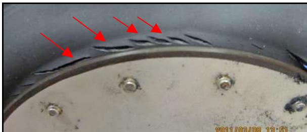
Figure 5: Internal diaphragm tear
